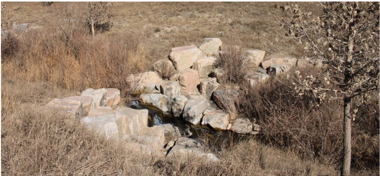
Figure 20 Rock drop structures not affected by submergence (November 2013)
