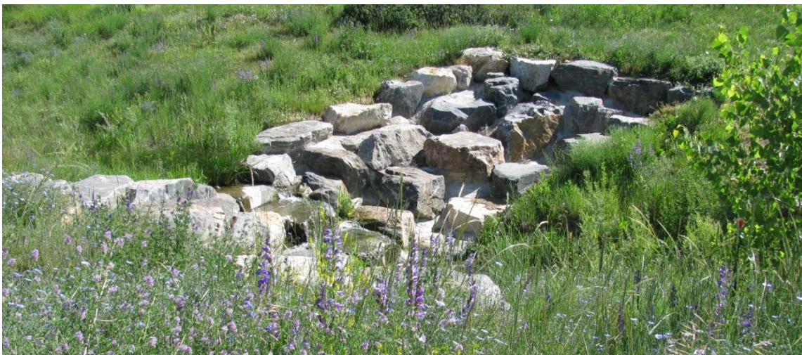
Figure 15 Check Dam from Figure 15 with Vegetation
