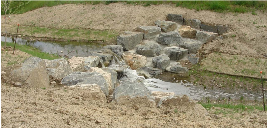
Figure 13 New Stone Check Dam Installed
