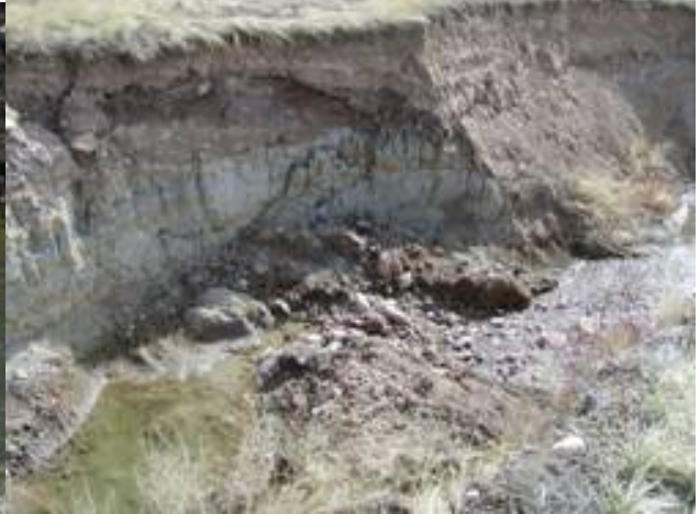
'04 Failing Embankment
