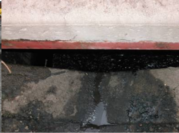
Pollutant Discharge Entering Storm Sewer
