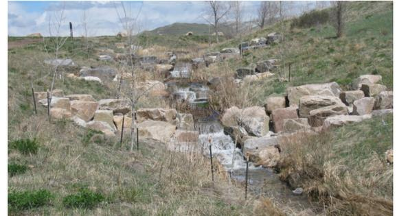
Park, which included 7 massive rock check-dams and new vegetation. Coyote Gulch revegetation began in June 2007 and became well established in 2008. The BCWA has a paired water-sampling program, which allows a determination on the effectiveness of the restoration effort at phosphorus
