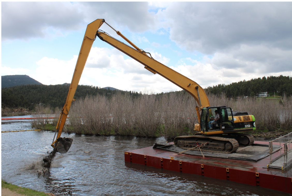
Figure 2 Dredge in Operation
