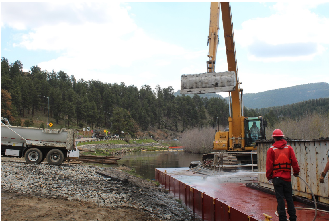
Figure 1 Staging Area and Dredge Barge
